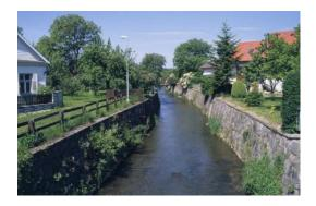
Figure 22: stone pitching tightly packed
